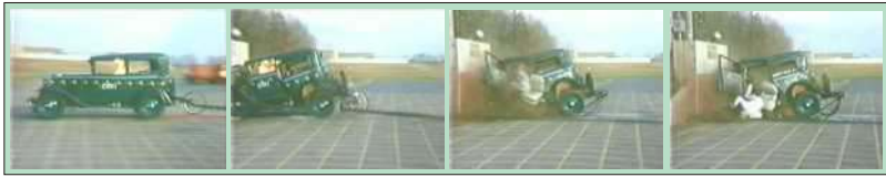
This model T's door opened in testing conducted almost 80 years ago.
